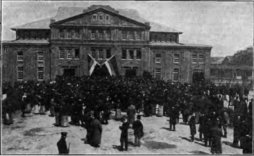
DELEGATES TO THE FIRST NATIONAL ASSEMBLY OF CHINA AND THE ASSEMBLY HALL
