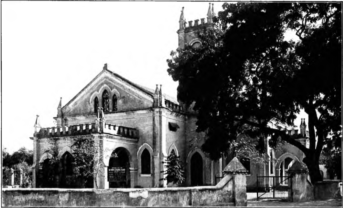
THE METHODIST EPISCOPAL CHURCH AT LUCKNOW, INDIA
