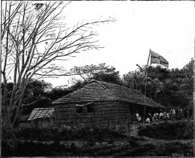
COMBER MEMORIAL STATION.—MR. LEWIS'S HOUSE. (From a Photograph.)
