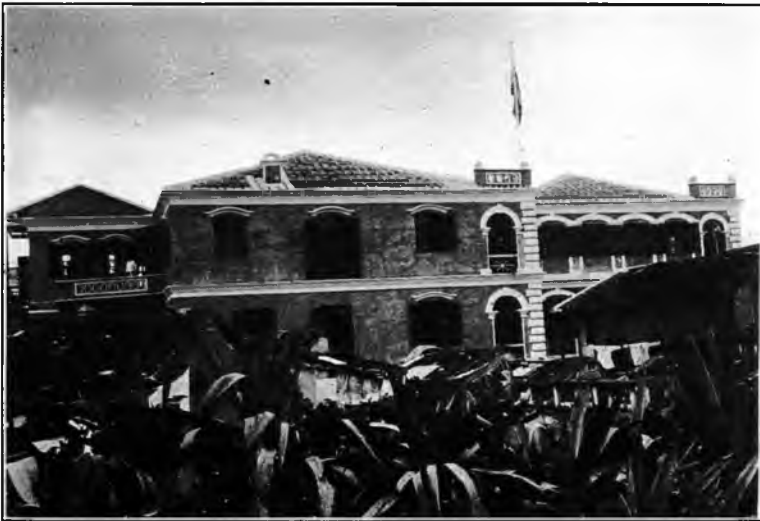
The new Sin-koe-a School Building distant side view.
